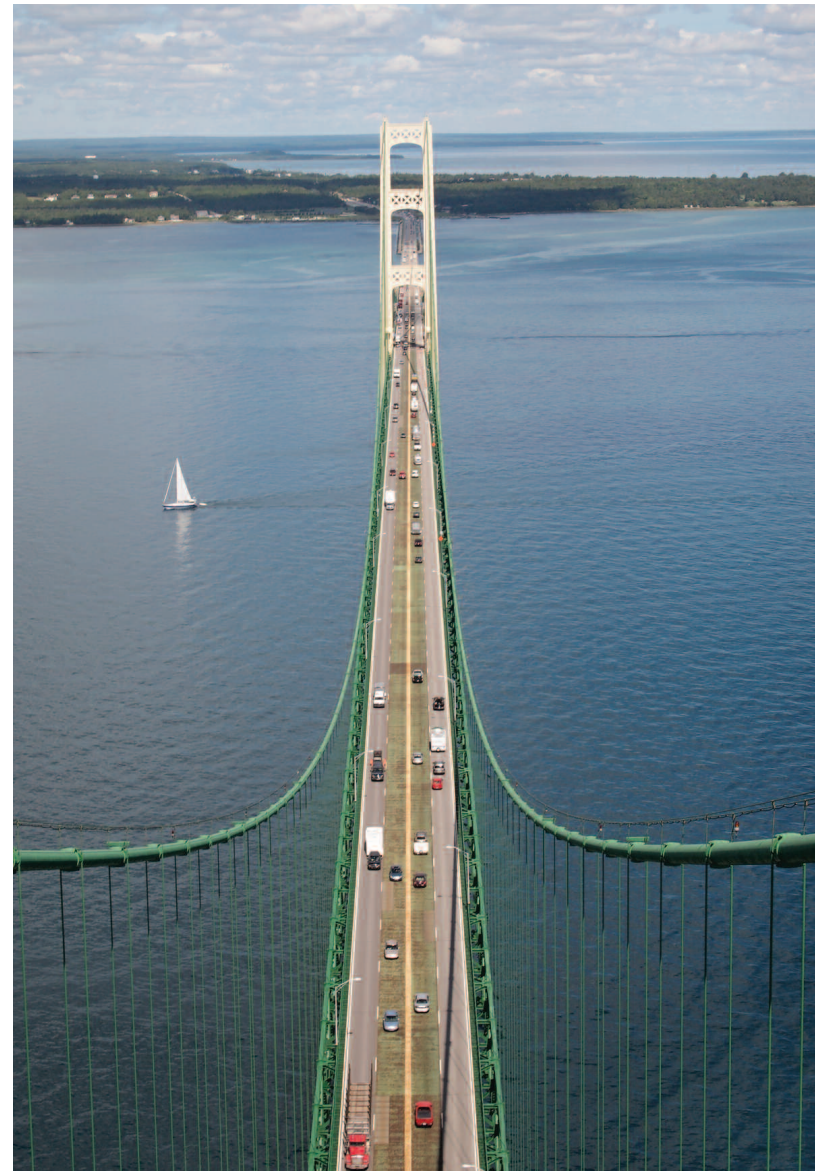
On Labor Day, thousands will enjoy the thrill of a lifetime by strolling the Mighty Mac. During peak summertime season, the bridge transports more vehicles across the Straits of Mackinac in a single month than the ferry system did in an entire year when it was in operation. PHOTO BY JIM AKANS
